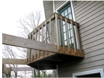
Upper, Balcony Deck
